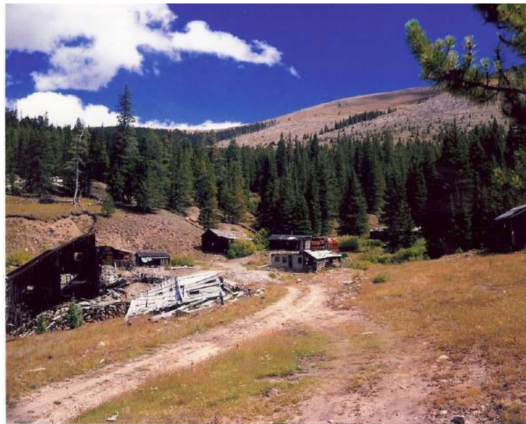
Laurim mill and shop buildings, ca. 1960
