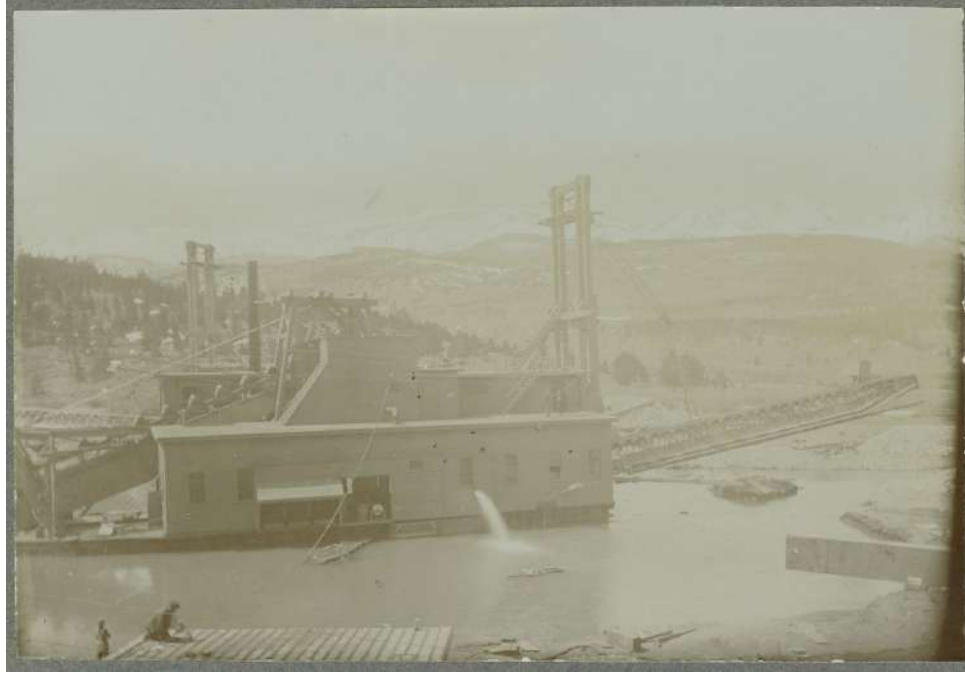
Reliance dredge in French Gulch, 1906
