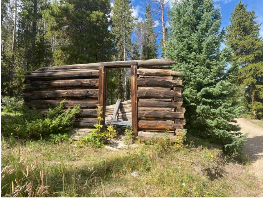
Top-priority cabin, currently strapped together to prevent collapse
